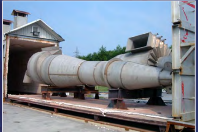
Heat Curing and Post Weld Heat Treating of Refractory Lined Cyclones
