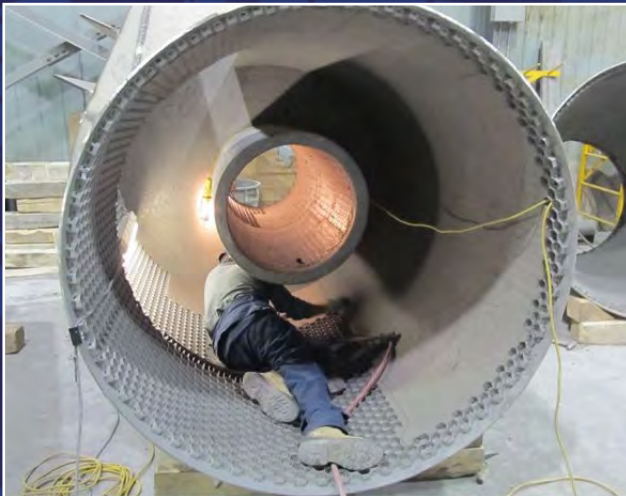
Installing Refractory Lining
